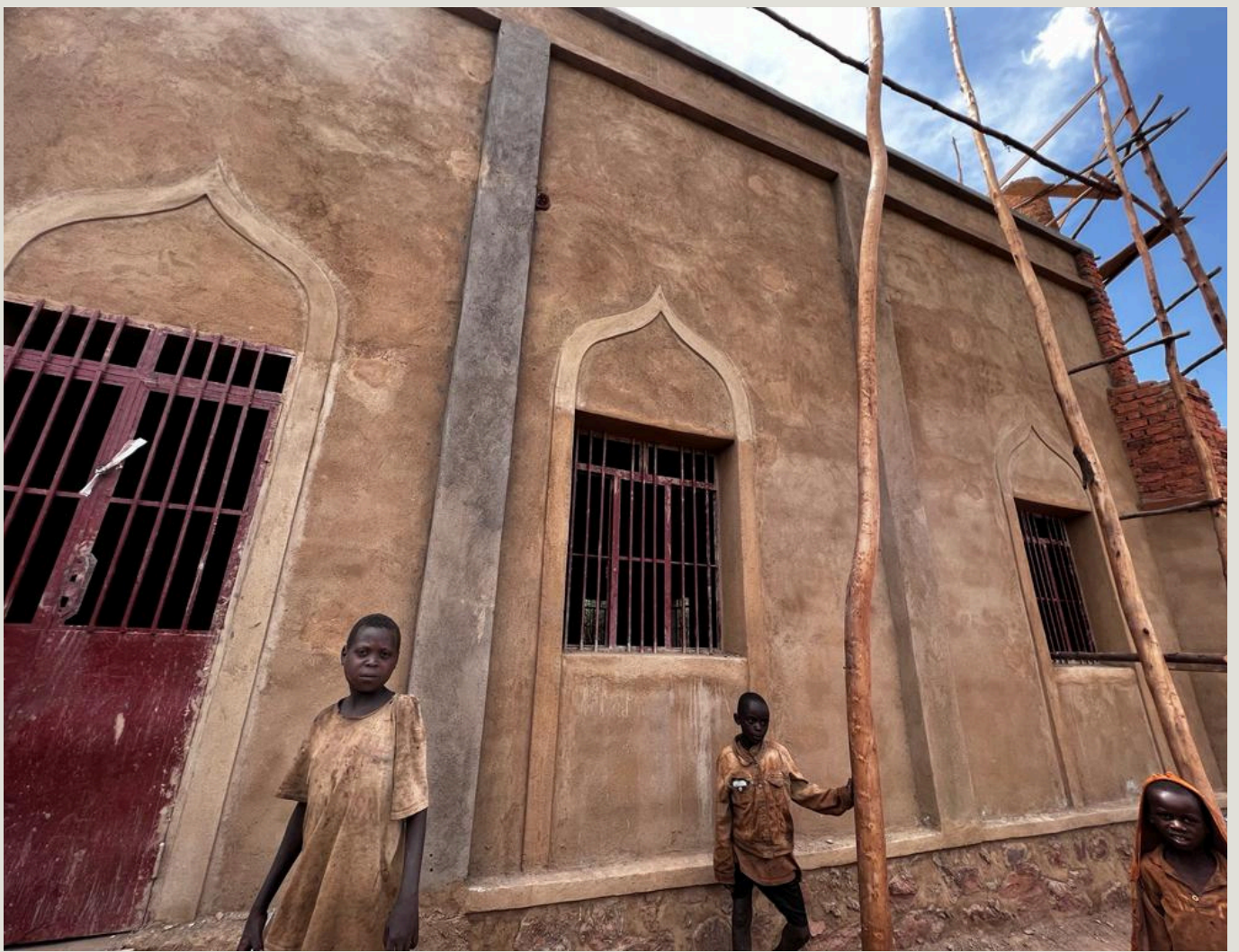
Picture - Masjid in Burundi under Renovation
