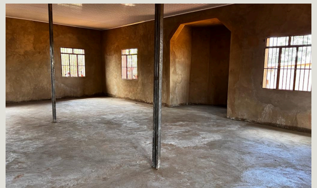
Picture - Renovation in progress
